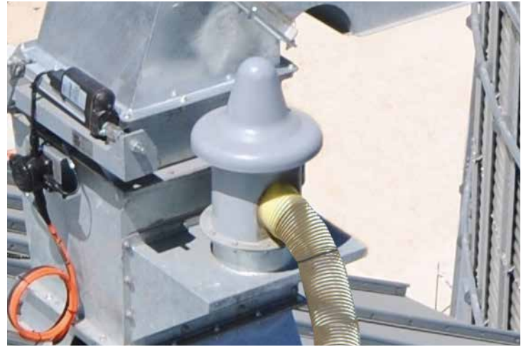
Silo top at the moment of overpressure relief through VHS-C membrane-type valve
